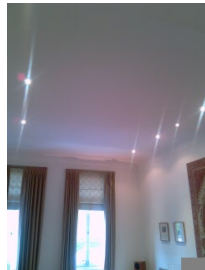
All of Ceiling to Room, Ceiling Finish, Mouldings, spot lights (6)
