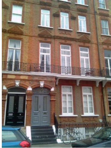
Front of building
